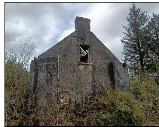
Plate 4-21 Vacant property 4 - south aspect
