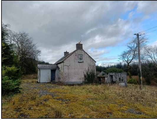
Plate 4-16 Vacant property 3 south aspect
