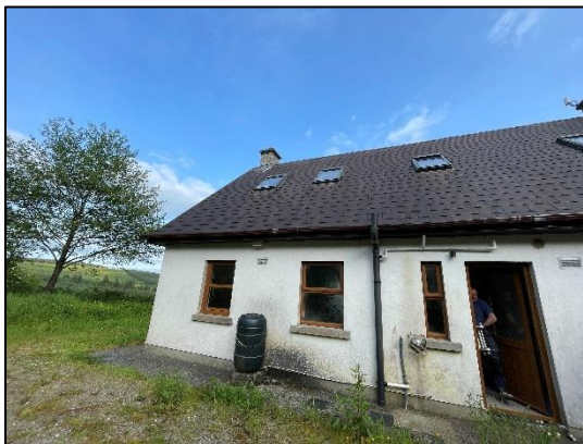
Plate 4-5 Concrete wall and slate roof
