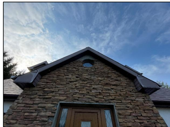
Plate 4-6 External stone wall cladding
