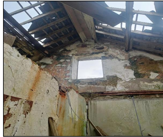
Plate 4-23 Vacant property 4 - Interior
