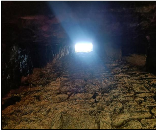
Plate 4-22 Vacant property 4 - Chimney stack
