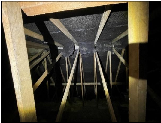
Plate 4-3 Underfelt in the attic
