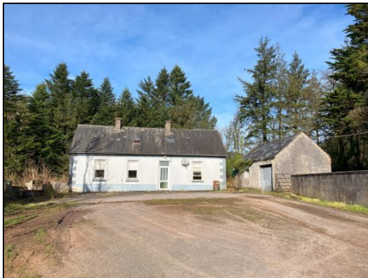
Plate 4-9 Main house and shed - High potential
